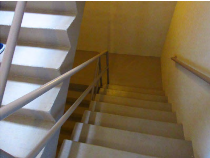
VIEW OF INTERIOR STAIRS
