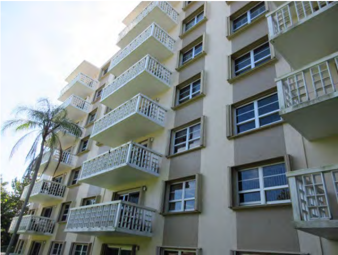
GENERAL VIEW OF BUILDING EXTERIOR FINISHES
