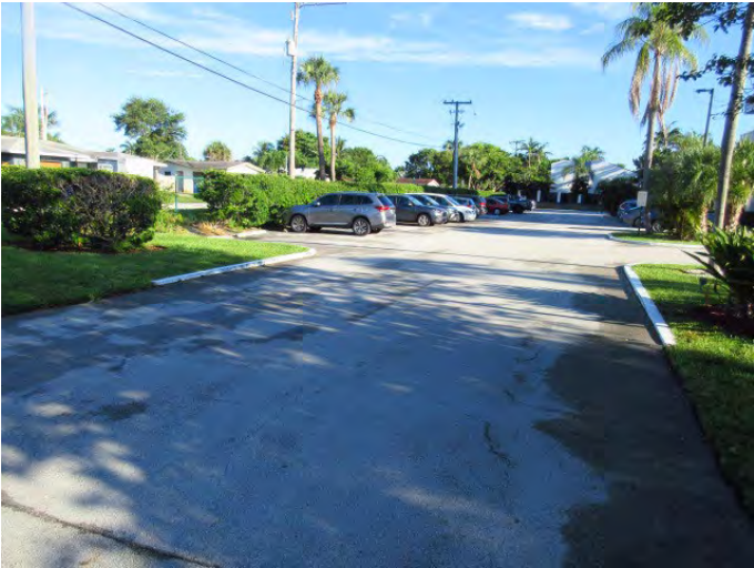
VIEW OF PARKING AND PAVEMENT
