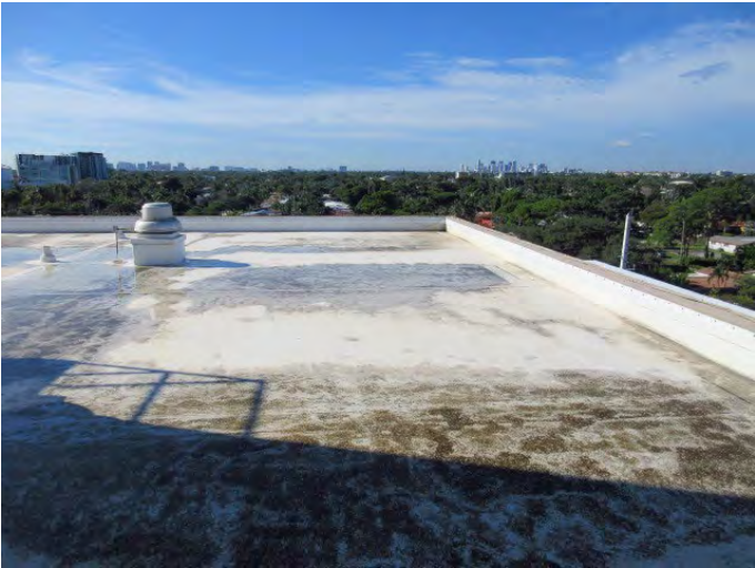
GENERAL VIEW OF ROOF COVERING
