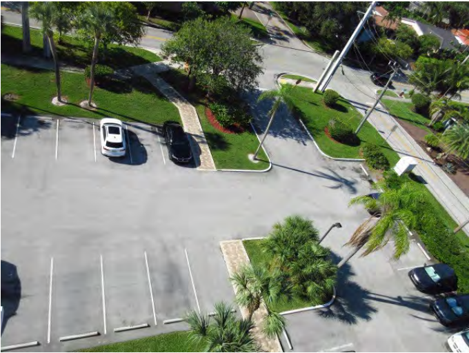
GENERAL VIEW OF PARKING AND PAVEMENT
