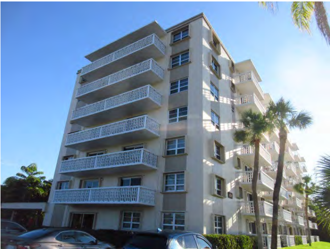
VIEW OF BUILDING EXTERIOR FINISHES
