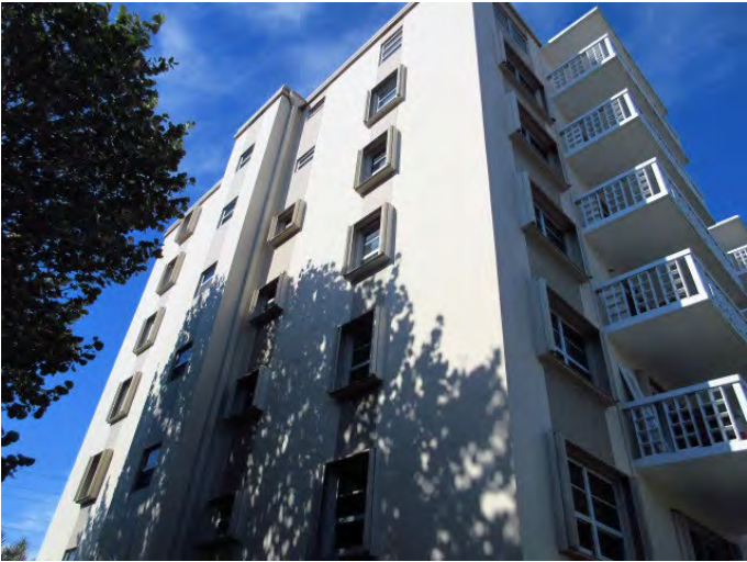
GENERAL VIEW OF BUILDING EXTERIOR FINISHES
