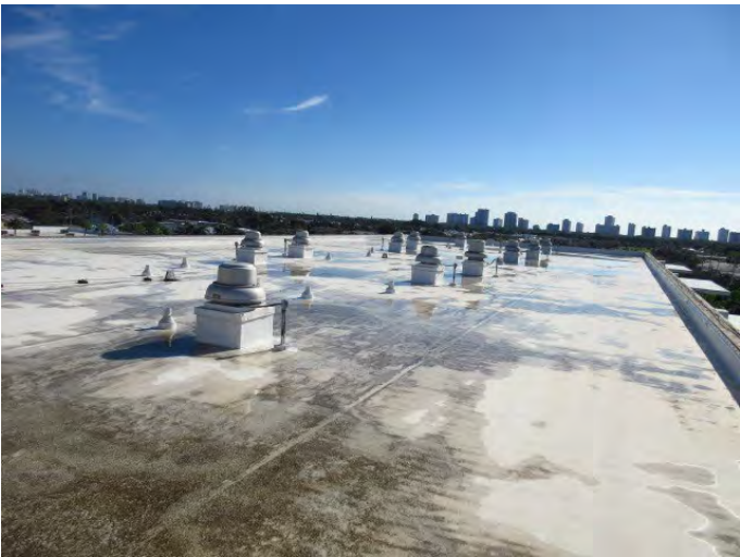
GENERAL VIEW OF ROOF COVERING
