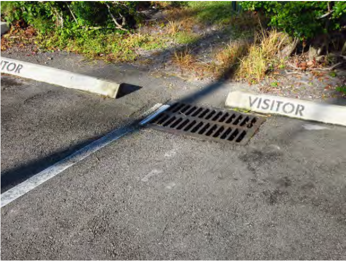
GENERAL VIEW OF STORM WATER INLET
